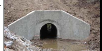
Upstream, the new culvert end was poured and tied-in to the existing stone arch.
