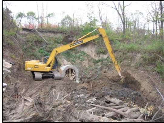
At the downstream outlet, an excavator clears room to pour an extension. Note the temporary trusses stabilizing the stone arch.
